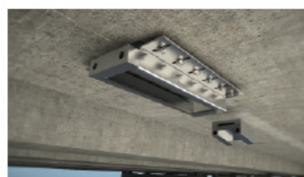
installing anchor block
