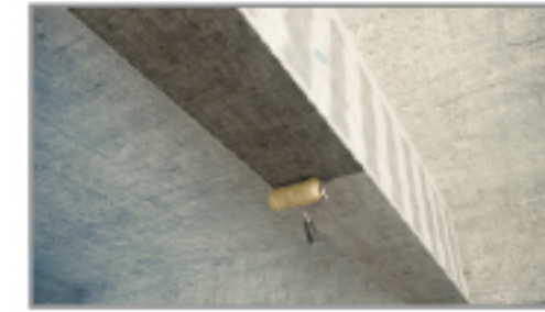
applying epoxy resin adhesive
