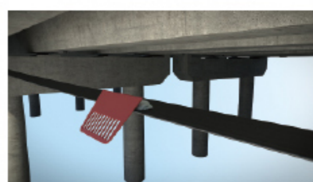
applying epoxy resin adhesive
