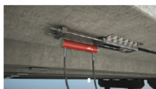
fixing jack and anchor bolt
