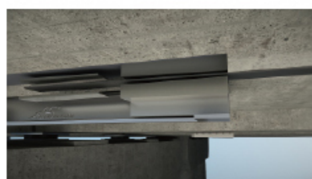
fixing carbon fiber laminate
