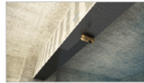
applying adhesive again
