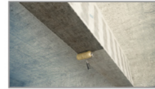
applying epoxy resin adhesive
