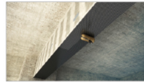
applying adhesive again
